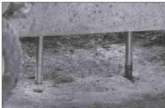
Fig. 8. Stone, with pins, offered to drilled holes. (© Alan McKinney.)
